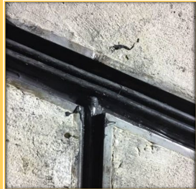
SF225 seal "T-spliced" into SF400 seal
