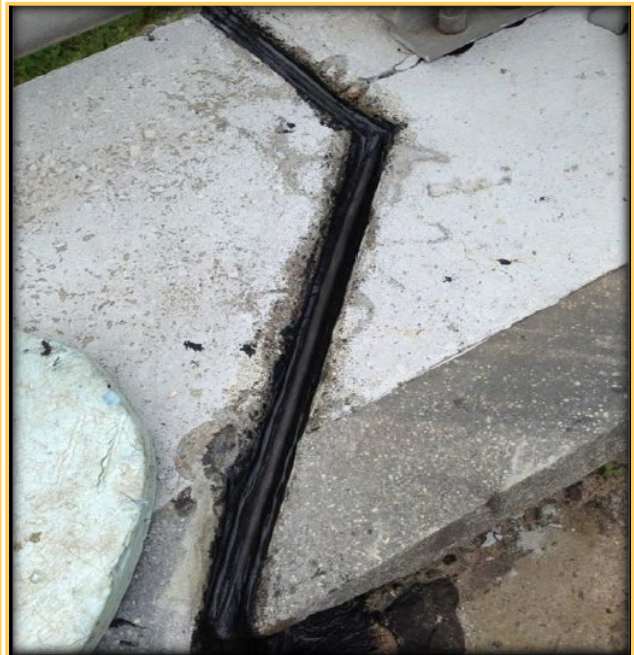
SF225 seal spliced to accommodate a skew
