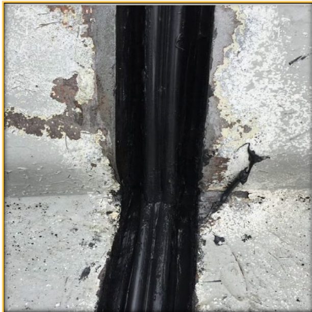
SF400 seal spliced to turn up a barrier wall
