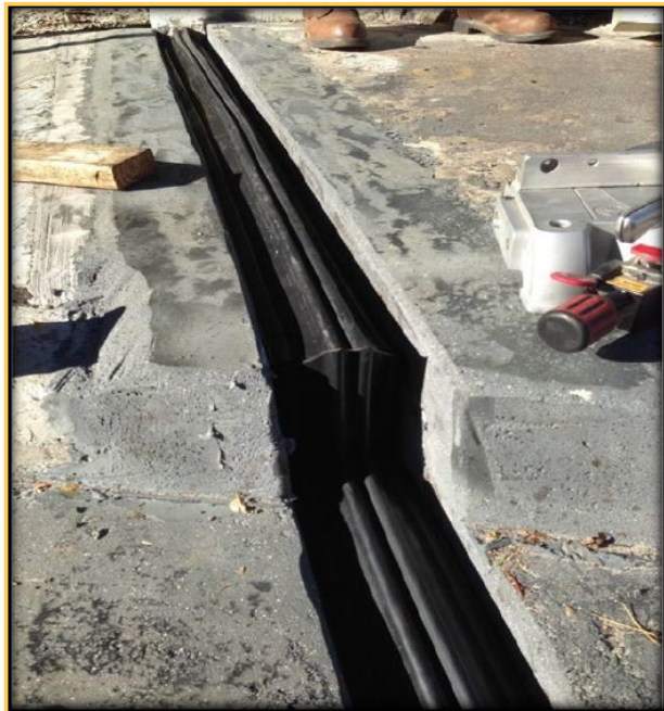
SF500 seal spliced to transition from road, up curb, and into sidewalk
