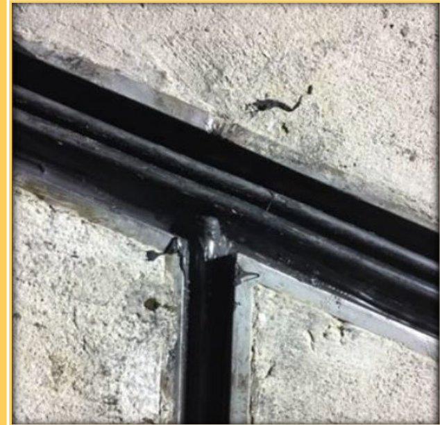
SF225 seal "T-spliced" into SF400 seal
