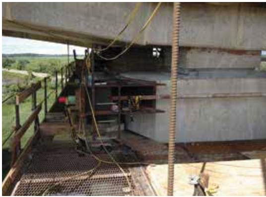
Pier column compression collars.
