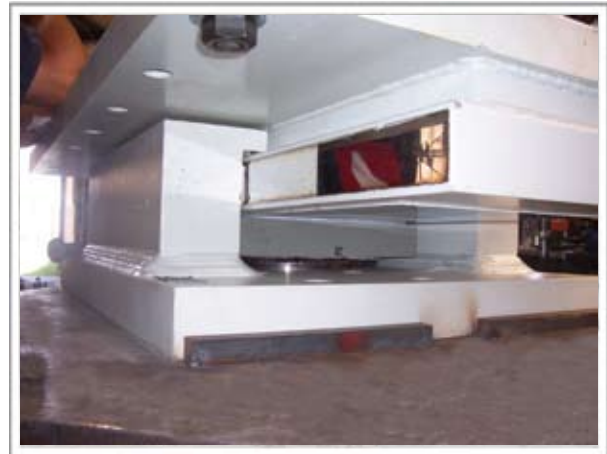
North Arm Bridge, Vancouver, BC Canada
